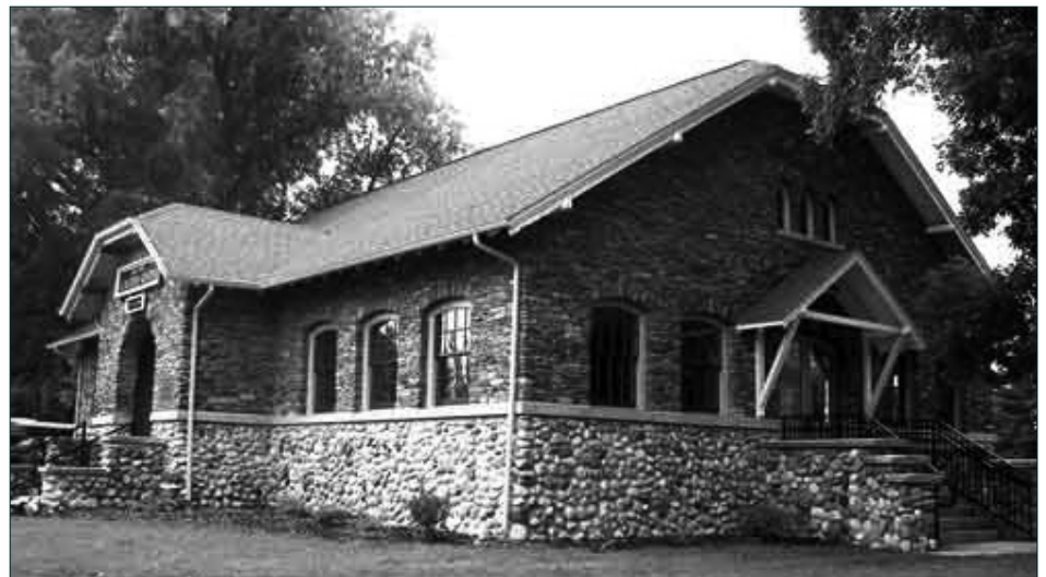
Beall Park Arts Center is the restored home of William and Rosa Beall, early Bozeman settlers and co-founders of the city. It sits on 2.2 acres of park, converted from their farm.
